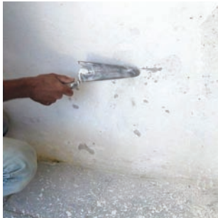
Clean the wall of dirt and dust.
