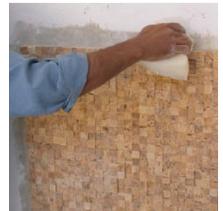
Wipe excess material from all edges.
