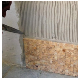
Remove excess material around tiles.
