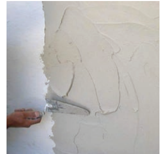
Apply the mortar evenly.
