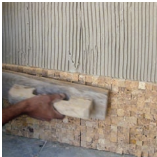
Press tiles together for a good hold.
