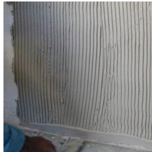
Make necessary adjustments to prevent mortar from spilling.
